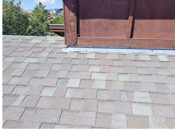
Metal flashing in good condition.
