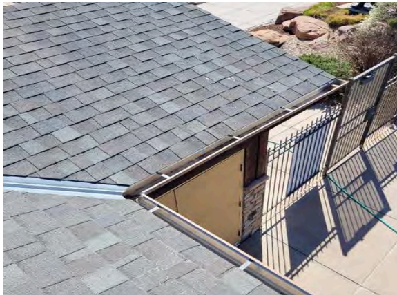
All gutters in good condition.
