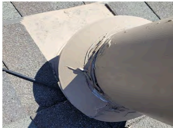
All penetrations in good condition.
