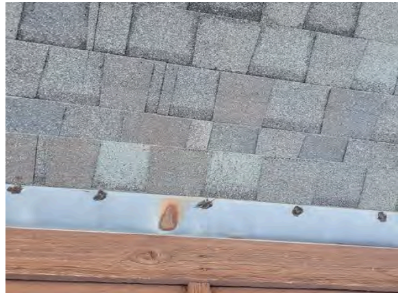
Metal flashing in good condition.
