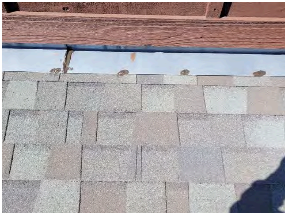
Sealed all exposed nails.
