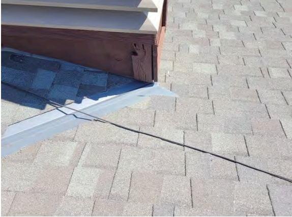
Metal in valleys is in good condition.
