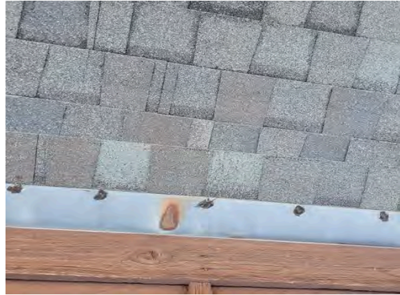
Sealed all exposed nails.
