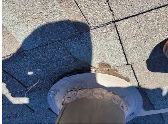
All penetrations in good condition.
