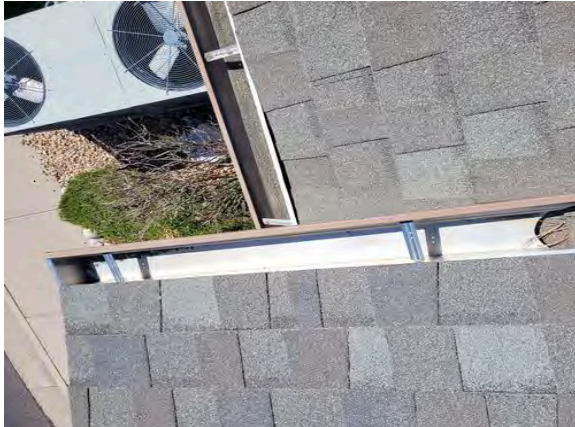
Gutters are in good condition.
