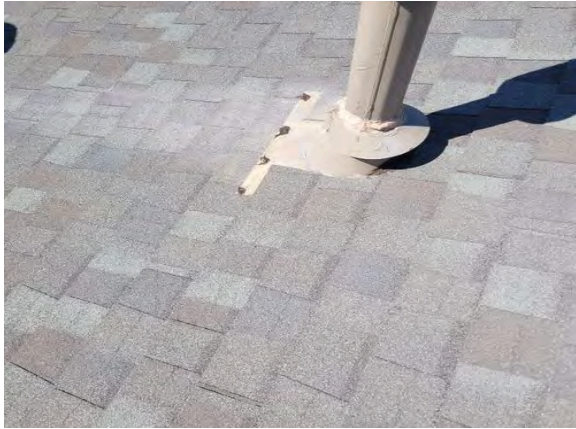
All penetrations in good condition.
