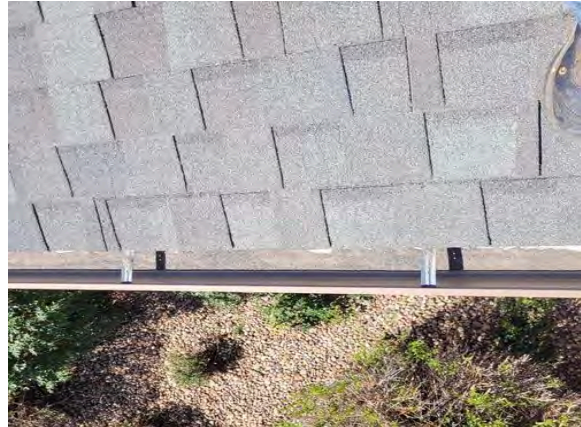
Gutters are in good condition.
