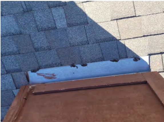
Metal flashing in good condition.
