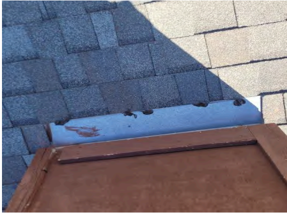
Sealed all exposed nails.
